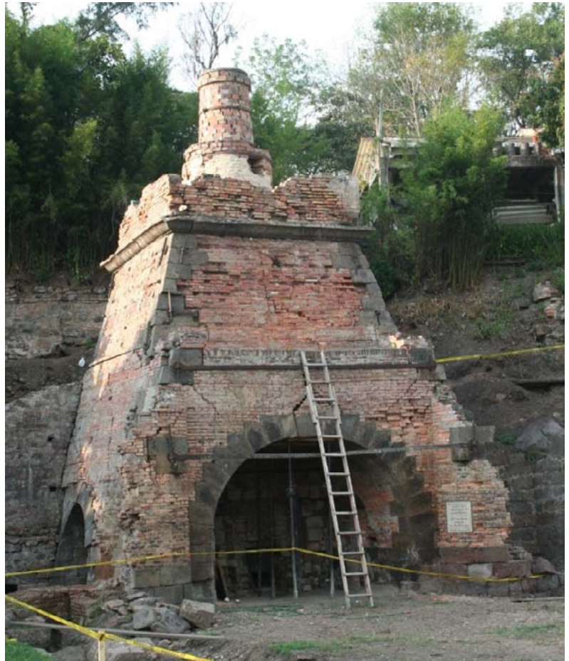
The masonry blast furnace at the Ferrería de Pacho ironworks in Colombia. At the top of the 9 m pyramid was a terrace around the chimney and the charge door of the furnace. A bridge connecting it with iron ore, charcoal and chalk store. See page 6.
